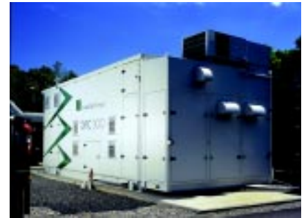
FuelCell Energy's first commercial product, the DFC300A, produces 250 kW
